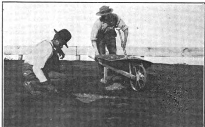
Filling the soft spots and making the surface hard and level
